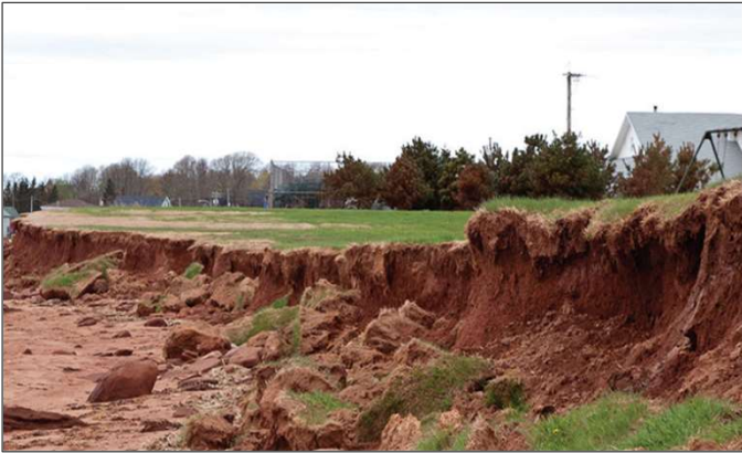
Figure 1. Example of bank erosion at Victoria Provincial Park
