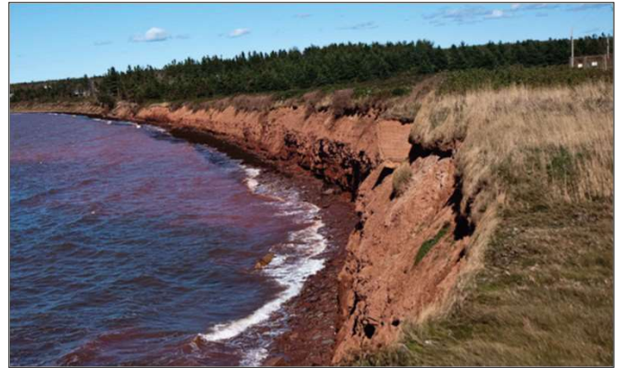
Figure 2. Example of cliff erosion at Cape Egmont
